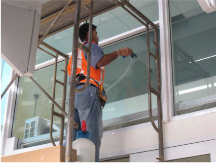
Installation of 3M Ultra Security
